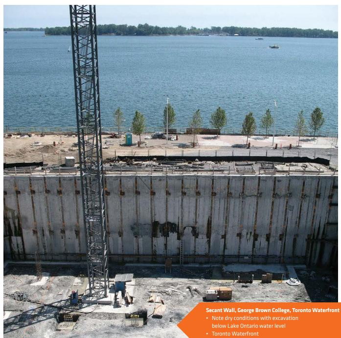
• Secant wall supported by rock anchors
